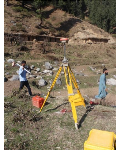
Figure 4: Topographic survey of Gabeen Jabba underway
